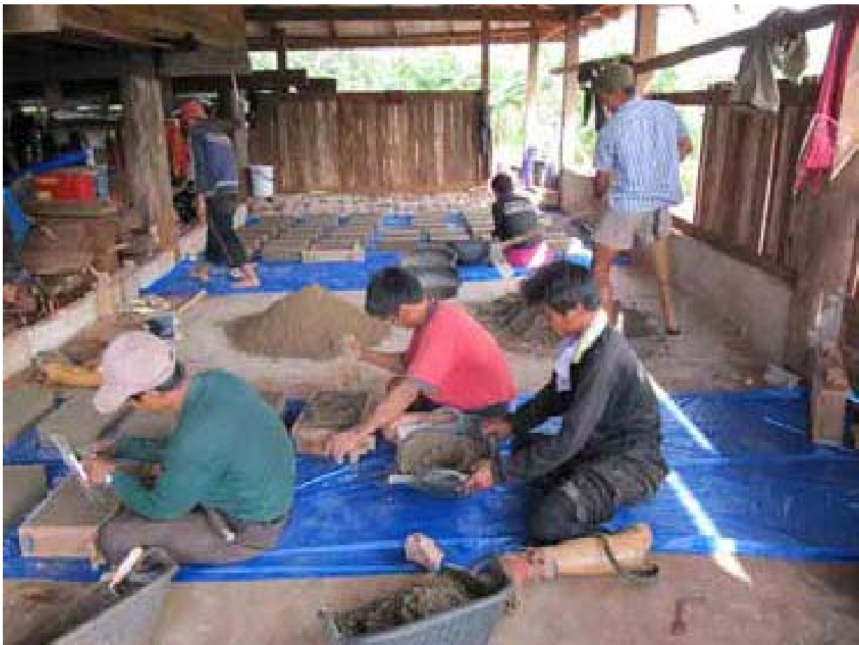
Training to make concrete blocks
